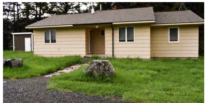
The newly remodeled Resident Manager's house.
